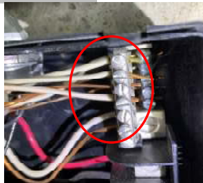
Neutrals/ grounds not separated in sub panel
