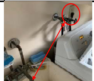
Outlet is not GFCI protected
