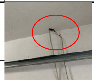
Extension cord wiring
