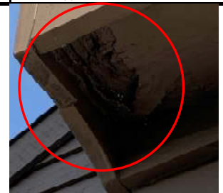
Damaged soffit (South)
