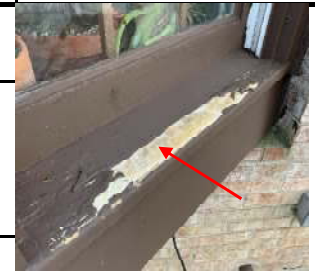
Moisture damage and peeling paint
