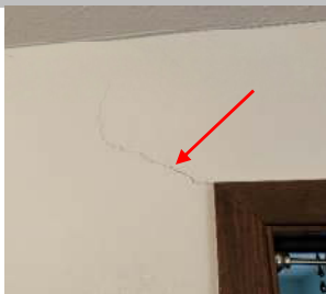
Cracking off corner of doorway
