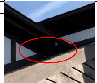
Missing downspout
