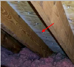
Frost accumulation on sheathing
