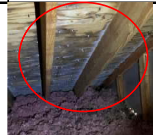
Frost and staining on sheathing in attic
