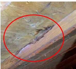
Stains from old leaks in garage attic
