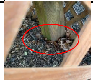
Main posts in direct contact with soil
