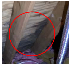
Moisture staining on sheathing
