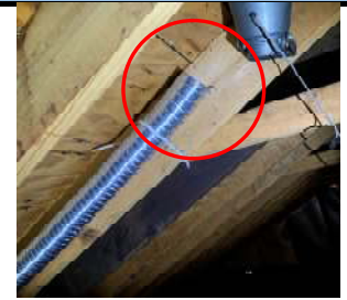
Bath exhaust vents into attic
