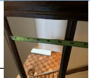
Baluster spacing is too wide
