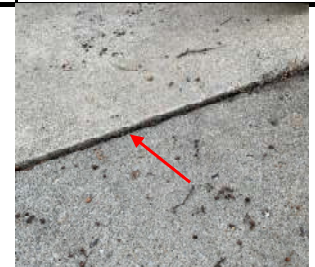
Trip hazard from settling
