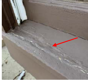
Moisture damage on window sill (North - bay)
