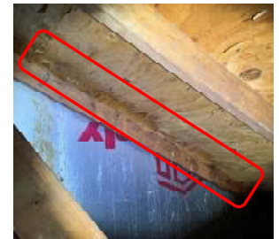
Moisture staining on sheathing
