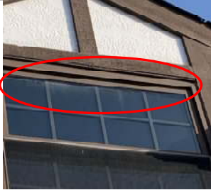
Possible fogged glass in window (South)
