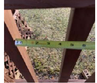
Deck railing balusters are too wide (recommend less than 4")
