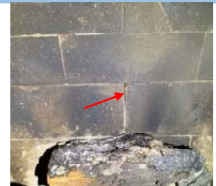
Open joints in firebox
