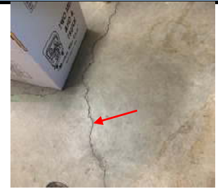
Typical floor cracks
