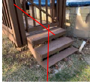
Recommend handrail on deck steps
