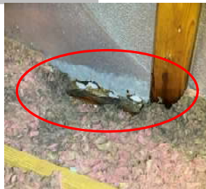
Moisture damage at sill in attic
