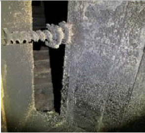
Soot/ creosote build-up in flue
