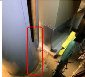
Relief valve extension is too short
